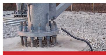
This anchor bolt installation shows an example of dangerous stress caused by too much height.
