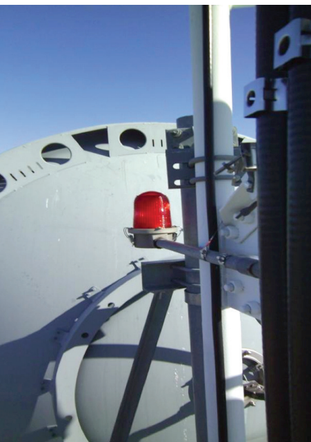
Picture 3: The FCC will allow an adjustment in the placement of an antenna with the proper filing, or the FAA (see AC70/7460-1K Chg 2) allows an adjustment in the placement of the lighting tiers by up to 10'. It is critical to understand that this is a 10' measurement from ground level, not to the base of the tower. Counting tower sections is not a safe means of measurement. All lighting must have an unobstructed view.
