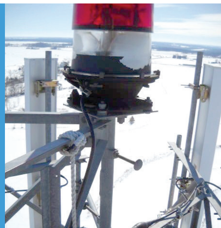
Picture 4: Note the crazed lens. Either the lens or the entire flashhead must be replaced.
