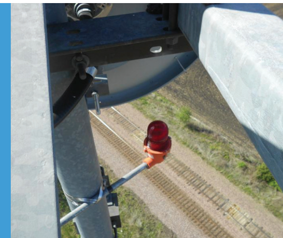
Picture 2: L-810 side marker light mounted behind antenna, creating an obstructed view.
