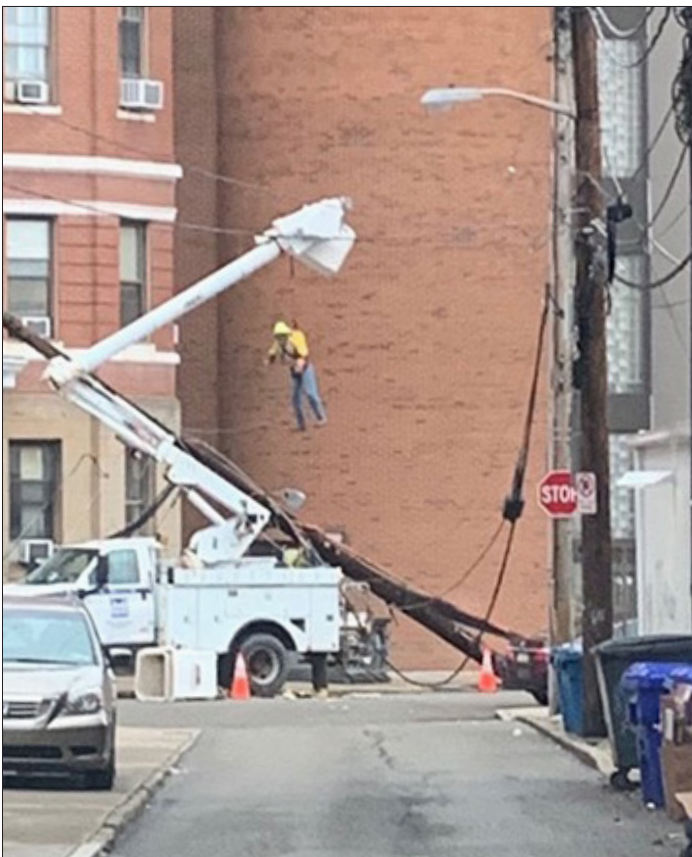
Proper fall protection is essential.
