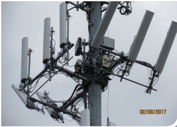
IMPROPER CANTILEVER
