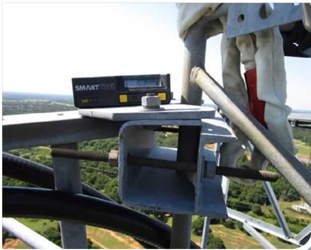
INCORRECT LEG SIZE FOR MOUNT
