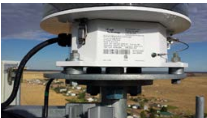
(Flash head leveling using washers as a spacer)
