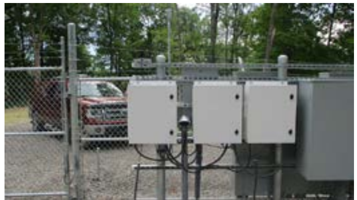
(Proper installation of photodiode/photocell at tower site)
