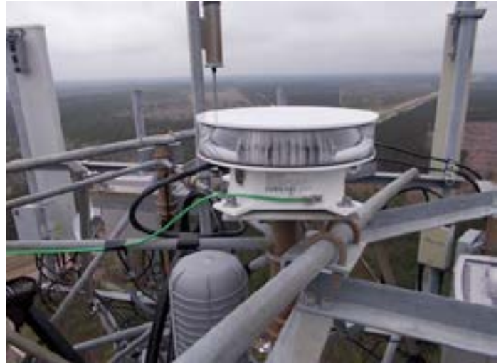
(Nesting of flash head within a several appurtenances at top of tower)
