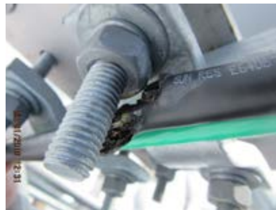
Cable rubbing against sharp edges, without proper spacing. (Cable damage due to rubbing across bolt and other sharp edges)
