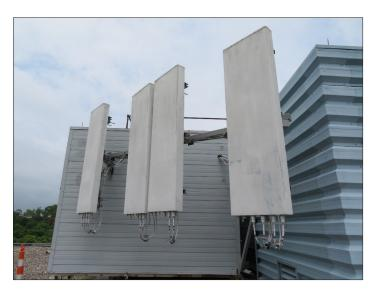
antennas located on the roof that are behind the ballast mount on which they are working. These antennas can be directional or omni directional exposing the employees to elevated RF fields. This includes the roof that they are working on, but also neighboring rooftops that are also on the same level. If possible, keep antennas above head level as the antennas will transmit over the head and not through the body.
