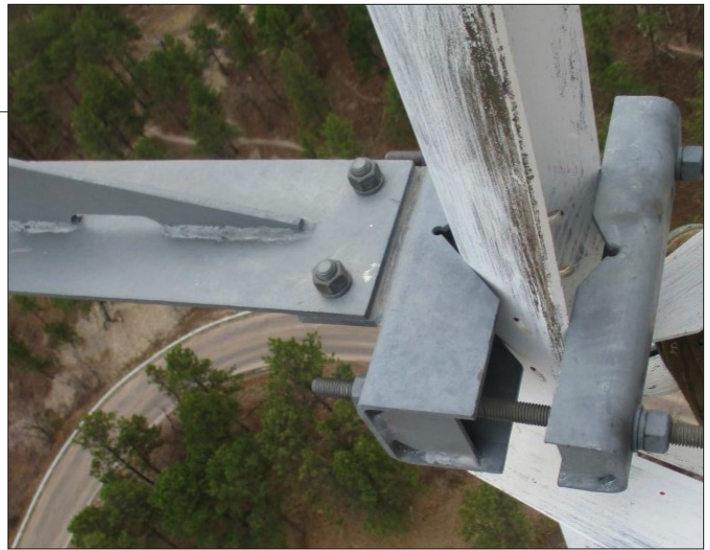
Mount-to-Tower Angle Leg
