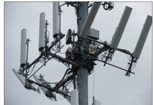
Figure 9 – T-Arm Mount Face Rotation
