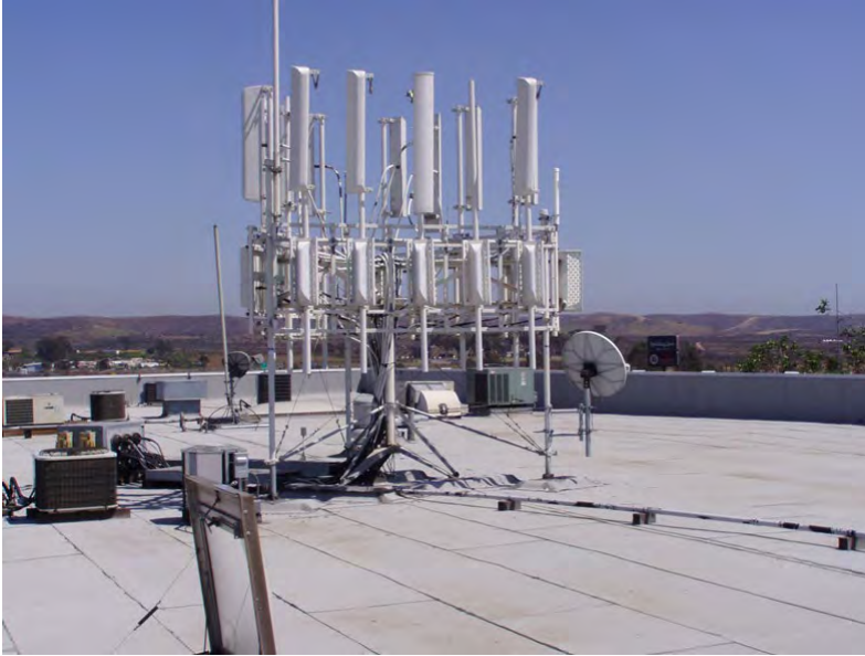
Figure A.b.3: Custom penetrating triangular frame with tripod mount
