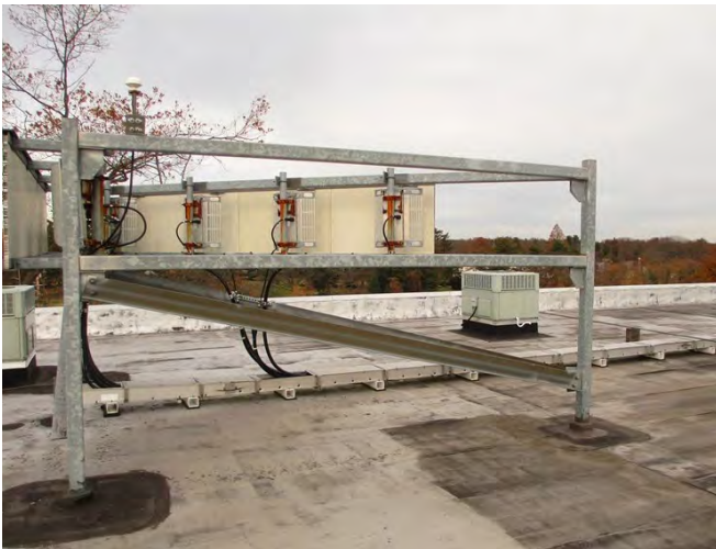
Figure A.b.2: Custom penetrating triangular frame
