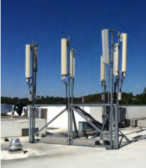
FigureA.b.7: Non-Penetrating ballasted triangular mount
