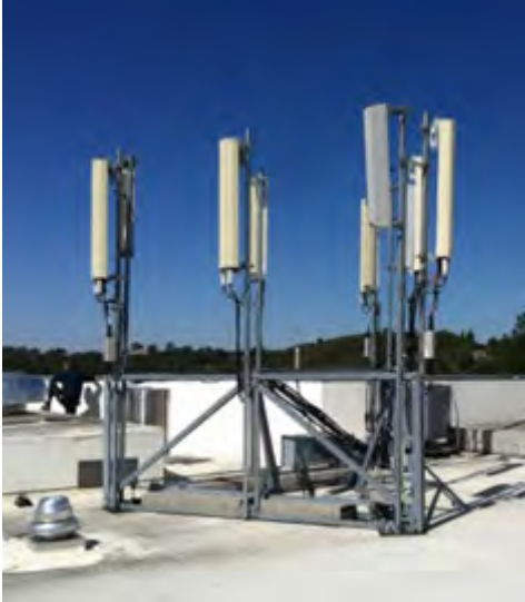
FigureA.b.7: Non-Penetrating ballasted triangular mount
