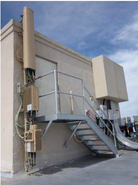
Figure A.a.2: Wall mount installed on the penthouse wall of a building
