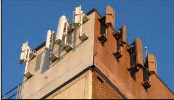
Figure A.a.1: Wall mount installed on outside of building
