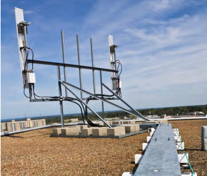
Figure A.b.5: Non-Penetrating ballasted sled mount
