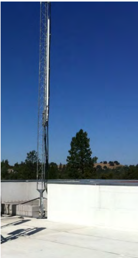
Figure A.d.2: Small Lattice Tower ballasted on corner of a building roof
