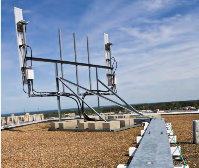
Figure A.b.5: Non-Penetrating ballasted sled mount
