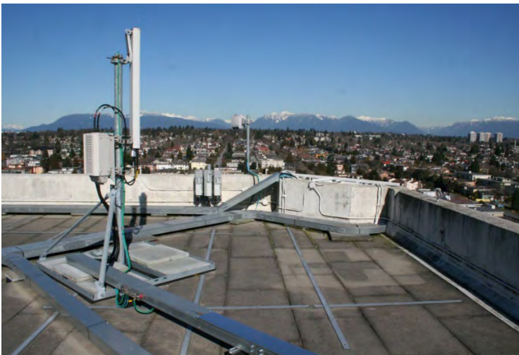
Figure A.b.6: Non-Penetrating ballasted tripod mount
