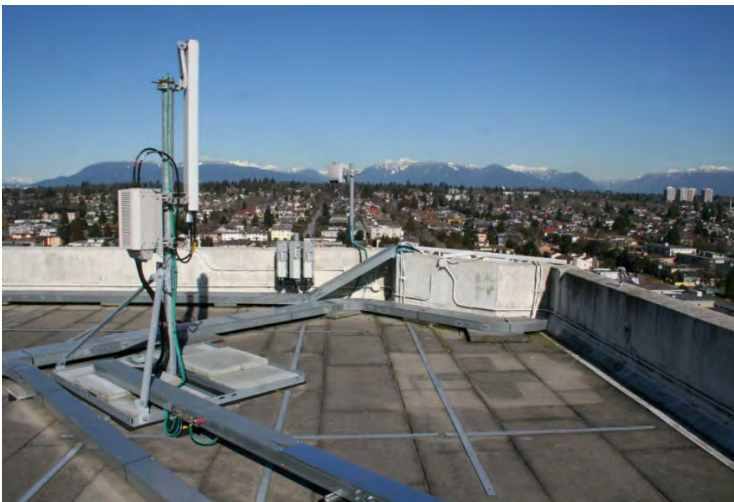
Figure A.b.6: Non-Penetrating ballasted tripod mount
