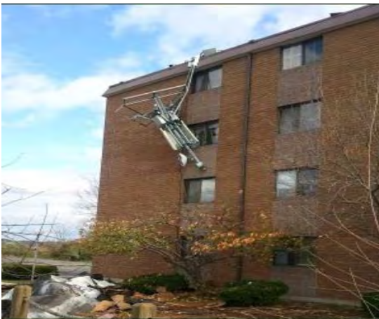
Figure B.3: Rooftop tripod mount fell off the roof as a result of not having enough CMU blocks or proper anchorage
