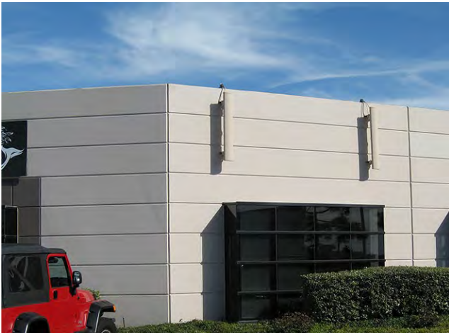
Figure A.a.5: Pipe wall mount installed on the wall of a building
