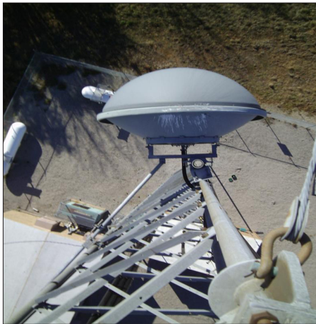
Figure 5: Improper Installation. In-board strut has too steep of a vertical angle, and the out-bound strut is improperly attached to the tower diagonal.
