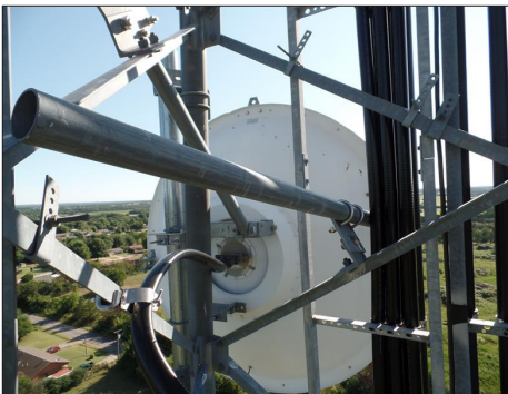
Figure 4: Improper Installation. The strut angle is too severe, and it is not mounted to the correct location on the microwave antenna. In-Board / Out-Board Struts with a Common Strut Support.
