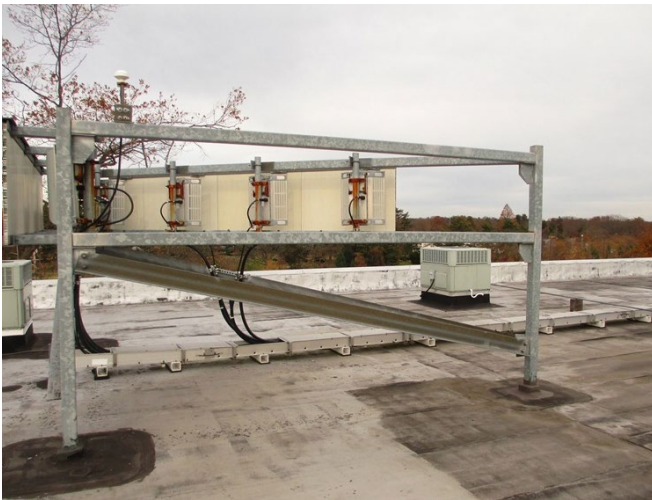
Figure A.b.2: Custom penetrating triangular frame
