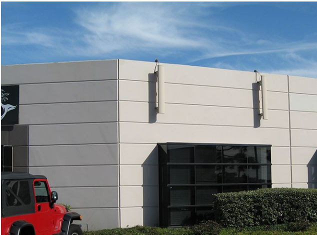
Figure A.a.5: Pipe wall mount installed on the wall of a building
