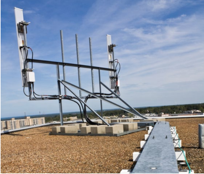
Figure A.b.5: Non-Penetrating ballasted sled mount
