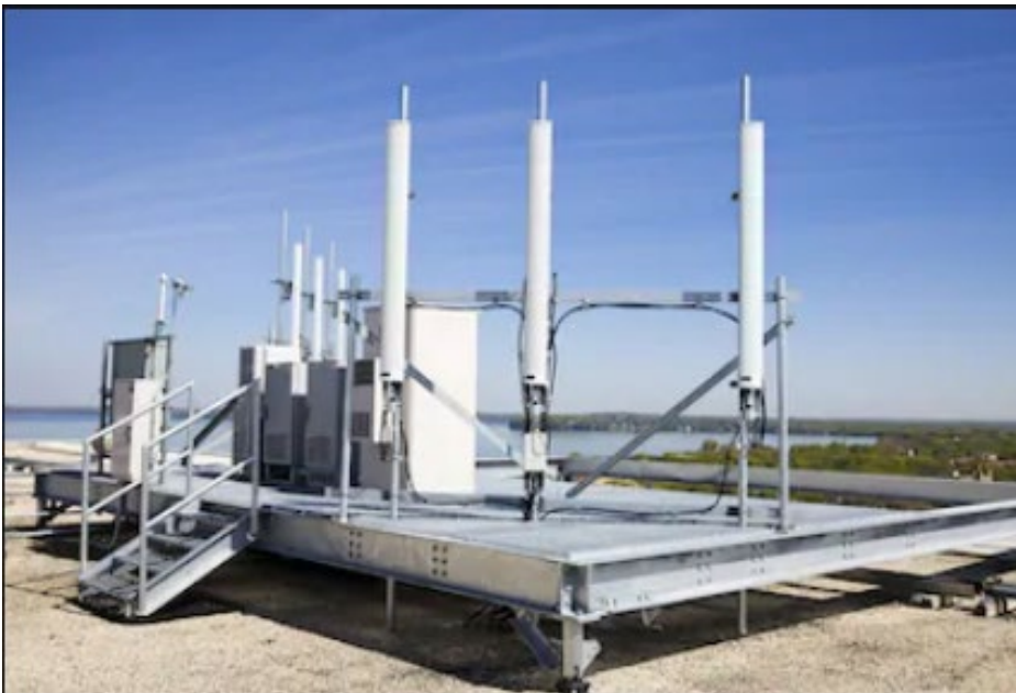
Figure A.c.2: Penetrating mount installed on equipment platform
