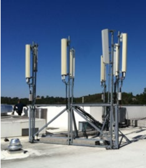
FigureA.b.7: Non-Penetrating ballasted triangular mount
