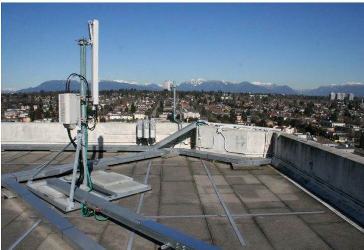
Figure A.b.6: Non-Penetrating ballasted tripod mount
