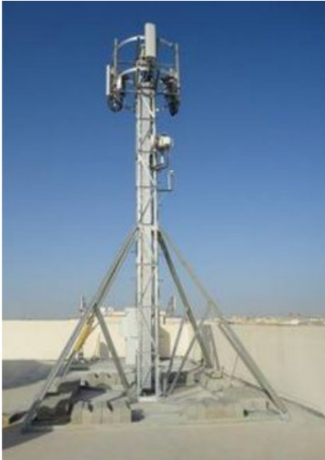
Figure A.d.1: Small Lattice Tower ballasted on corner of a building roof
