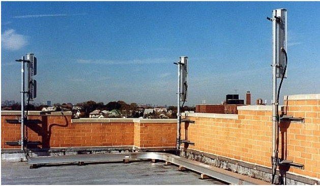
Figure A.a.4: Pipe wall mount installed on parapet wall of a building
