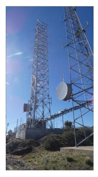
considerations are defined, then the focus moves to path design and identifying the "hub." The hub, which goes by many names, is where the microwave path needs to transport the backhaul to. Often this can be done with a single microwave path. A microwave path consists of two points with a microwave antenna (aka microwave dish) at each end, with at least one microwave antenna connected to the backhaul network. However, there
